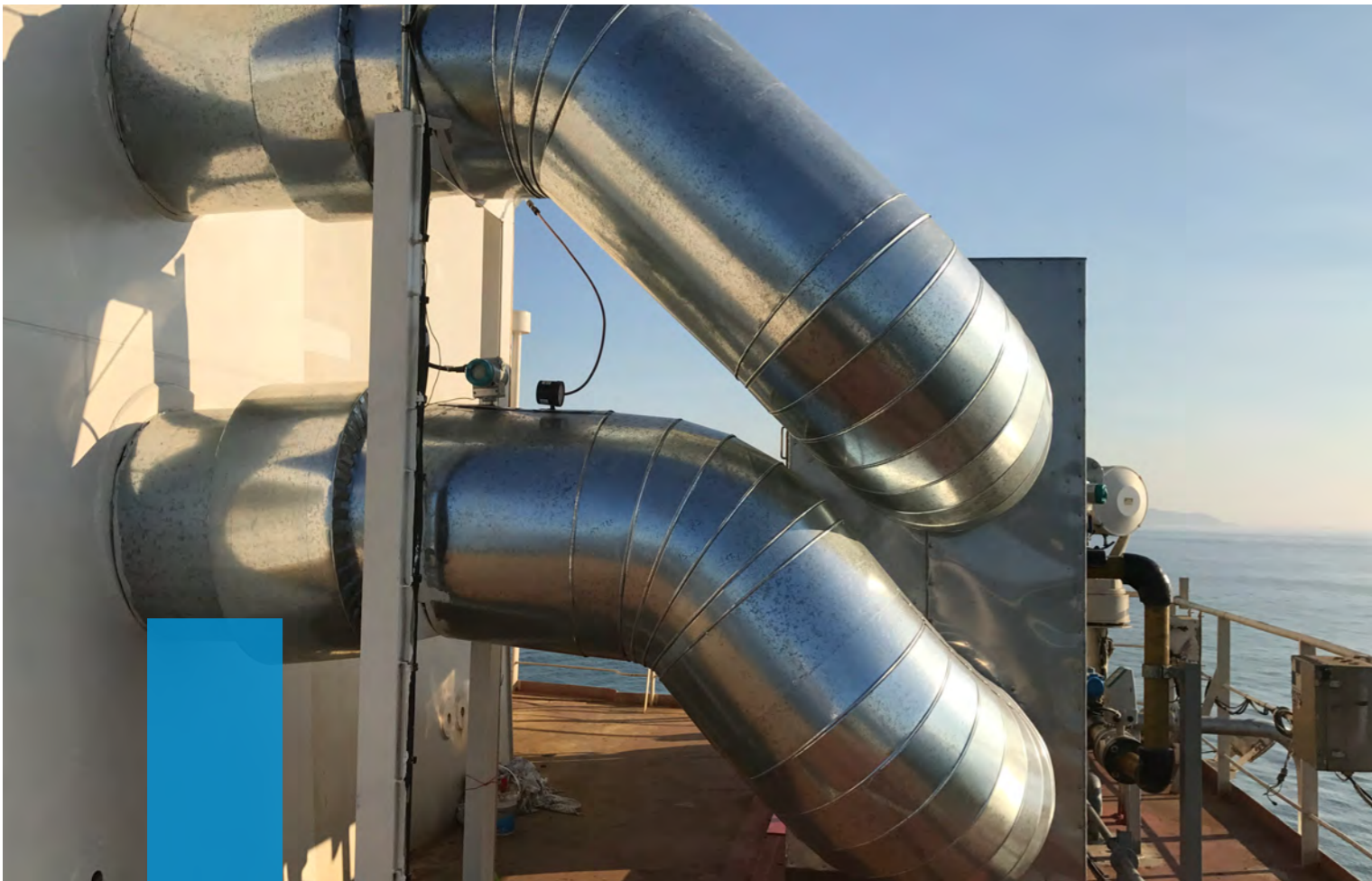
Viswa H-Scrubber – Simple connections in and out of the Exhaust Stack
